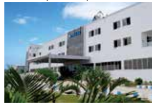
Rudrapur Plant (Green Building)
