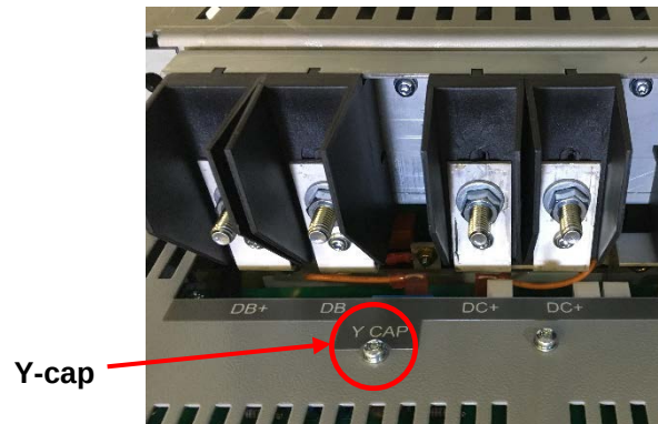
Top Terminal Area
