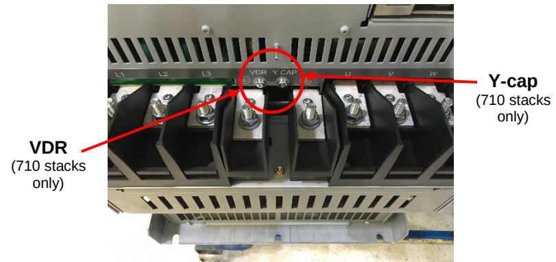
Bottom Terminal Area
