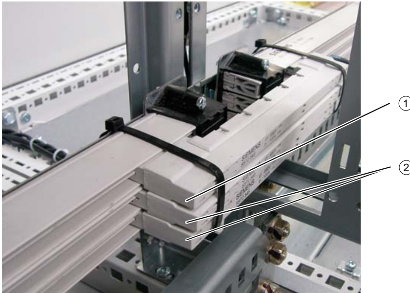
Figure 4-10 Connecting the auxiliary voltage busbar system when cabinet units are installed side-by-side
