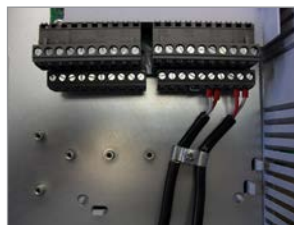
(b) Connection sample of the shield to ground
