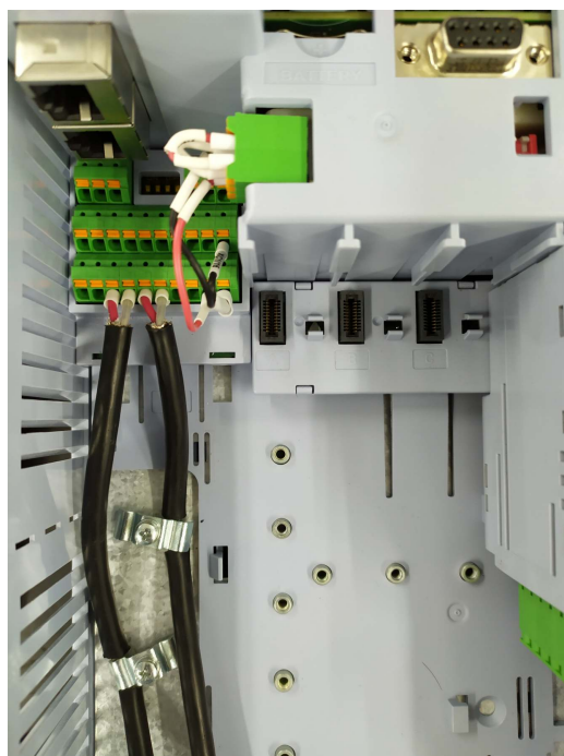
Figure 3.23: Connection example of control cable shield
